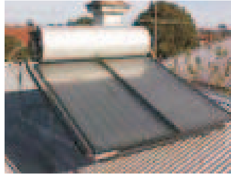
Figure 12.1 Solar Flat plate collector
