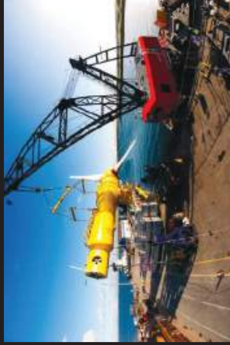
Deployment at EMEC
